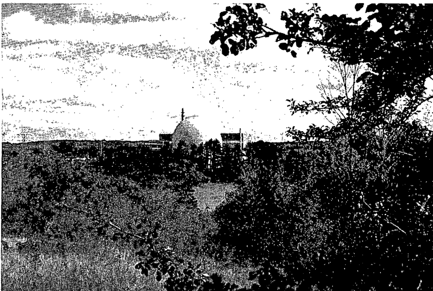
The Maine Yankee Atomic Power Company submitted a program to the NRC to correct and prevent the recurrence of deficiencies in administrative controls of its Wiscasset, Me., plant which had been found to permit development of unsafe conditions. NRC review of the program concluded that it was comprehensive, well conceived and properly implemented.
